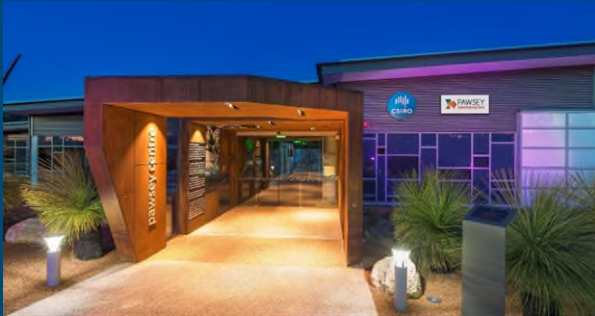
Figure 8 – Entry to the Pawsey Supercomputing Research Centre at Technology Park, Kensington WA
